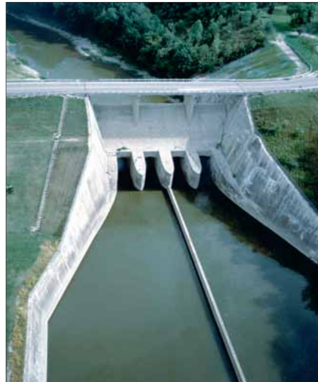
Taylorsville Dam near Vandalia is one of MCD's five flood protection dams.
