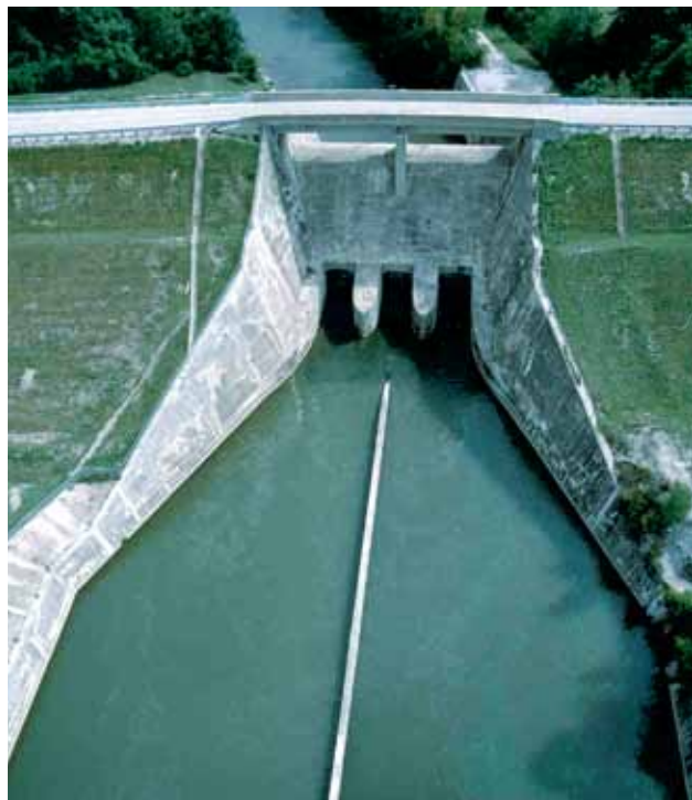
Huffman Dam near Wright Patterson Air Force Base is one of MCD's five flood protection dams.
