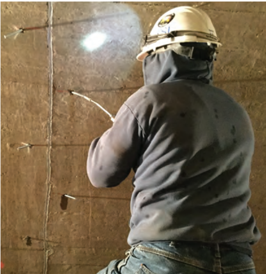
A worker injects polyurethane material to seal hairline cracks in the Germantown Dam conduit.
