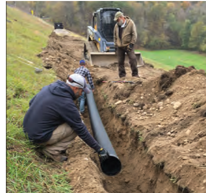
These collector pipes at Germantown Dam will reduce the potential for erosion.
