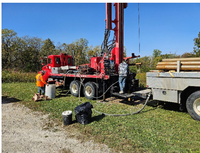
Installing a monitoring well at Eidson Woods Preserve.
