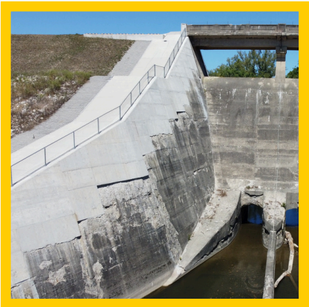
Restored concrete at Lockington Dam following completion of rehabilitation work.
